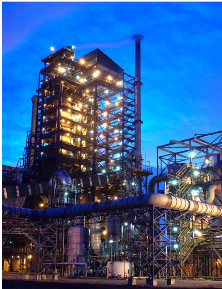
Figure 2 – The ISASMELT™ Plant at Mufulira Smelter
